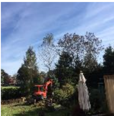
McParland Air spade work for Spruce and Cedar moves
